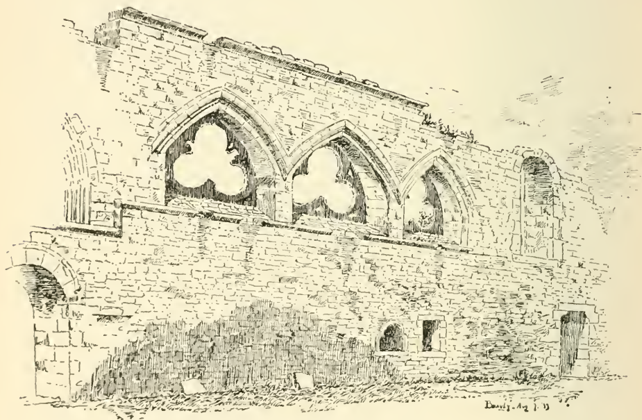
WINDOWS IN SOUTH WALL OF NAVE.
